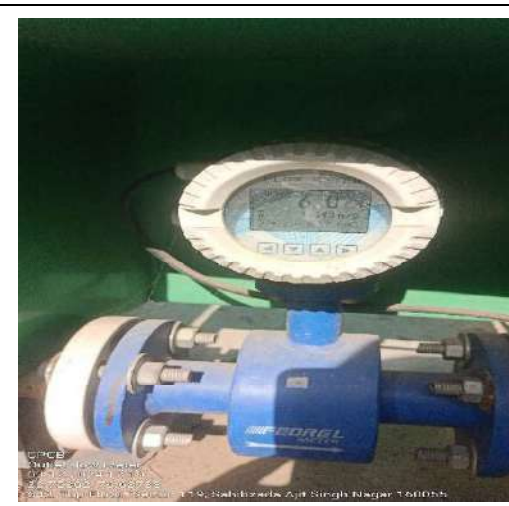
Outlet flow meter of 100 KLD STP, Sec. 119, Mohali
