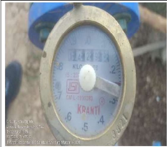
Borewell flow meter for Wellington Height housing 1&2
