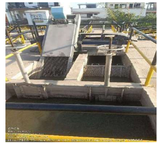
Manual & Mechanical Fine screen of 2.5MLD STP, TDI, Sec. 117, Mohali
