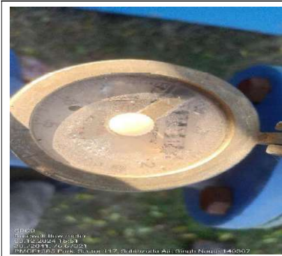
Mechanical Type Flow meter at Tubewell at Park of TDI, Sector 117, Mohali
